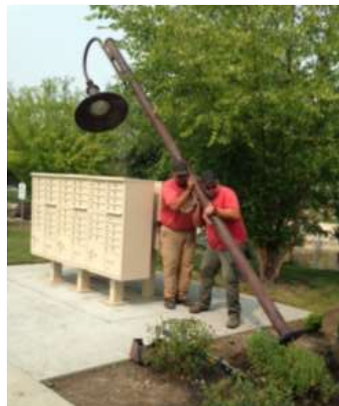
This light post was installed by Alloway Electric Co. workers above the cluster mailboxes on West Wildbranch Drive in the Waterview neighborhood.
